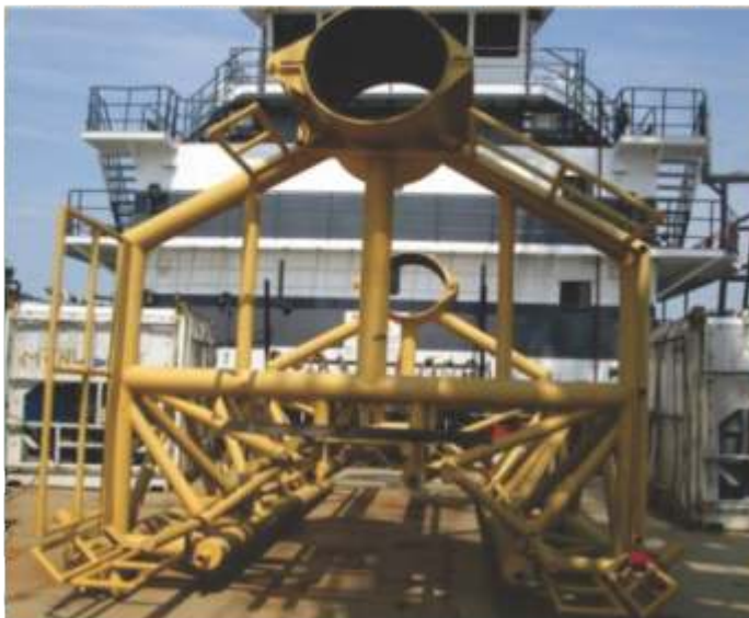
Top sides installation of Oron WS. KITA Marine &akam Boat Landings by STRUGA SERVICES LTD /ASCOT for APDNL
