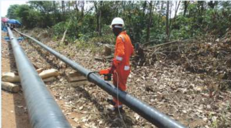
Holiday Detection Activity on 6" Gas Lift Pipelines X14KM in OML 124 for LNL/ADDAX Petroleum.
