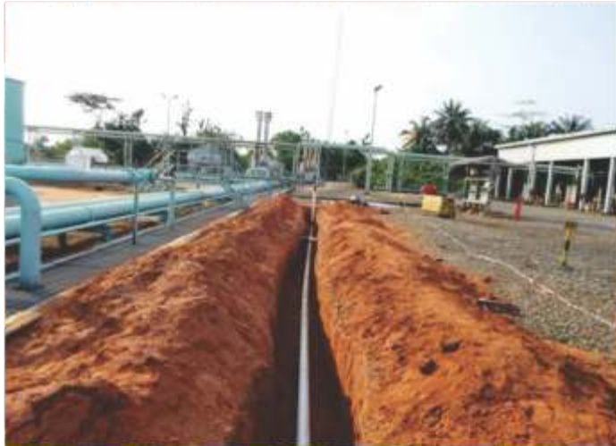
Piping fabrication and site Installation Of T-2500B Booster pump pipeline at Izombe Flow Station By STRUGA SERVICES LTD /ASCOT for Addax Petroleum
