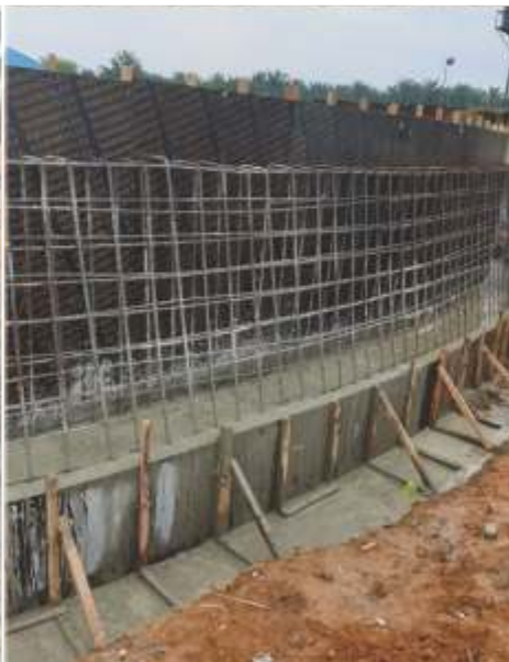
Construction of 26 Metre Diameter Tank Base Agwa Flow Station.
