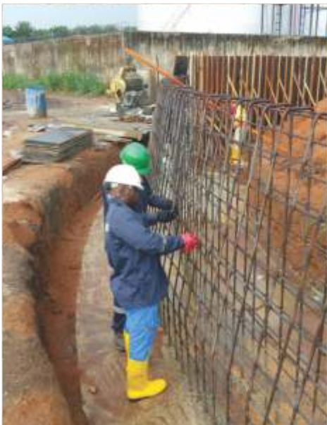
Construction of 26 Metre Diameter Tank Base Agwa Flow Station.
