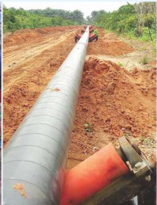
Holiday Detection Activity on 6" Gas Lift Pipelines X14KM in OML 124 for LNL/ADDAX Petroleum.
